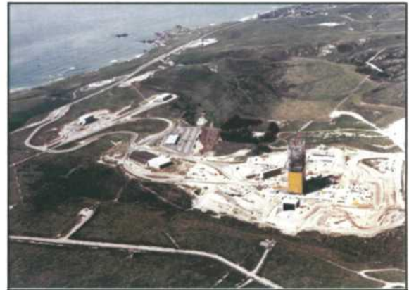
Construction of SLC-6 at Vandenberg AFB, CA - 1966
